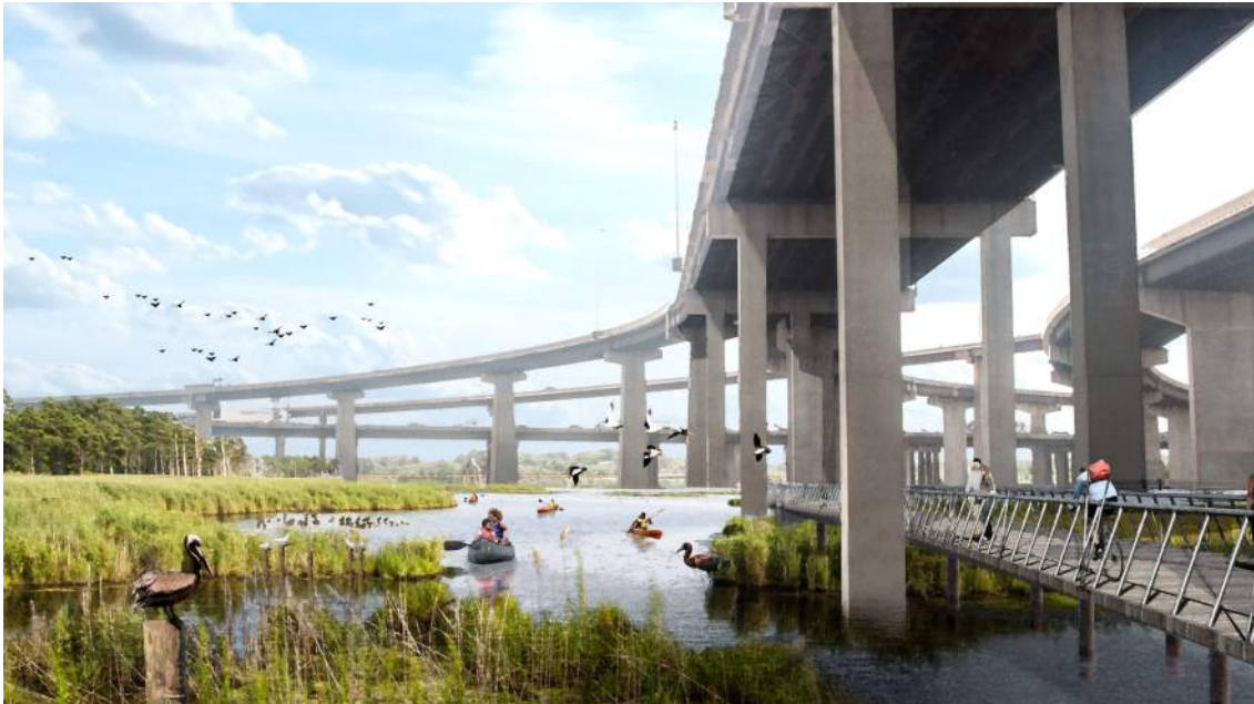
New wetlands and boardwalks will transform Ridgely's Cove into nature-based parkland. Credit James Corner Field Operations.
