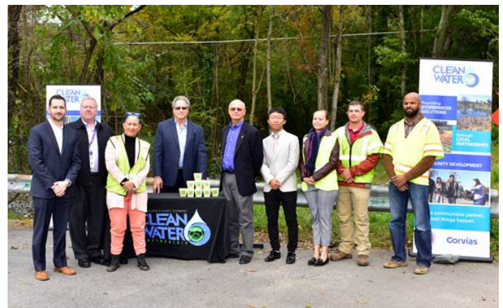
Figure 5-7. Representatives from Prince George's County, the Clean Water Partnership, the Low Impact Development Center, and the University of Maryland break ground on the new stormwater basin in Suitland, Maryland [27].
